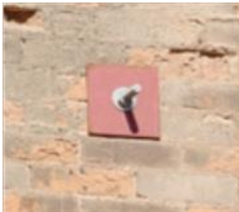
A steel plate with anchor bolts.
